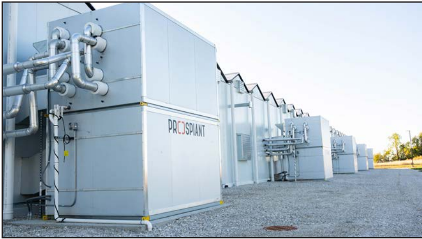
Example and schematic of Prospiant's Hydronic 4-pipe HVACD system
