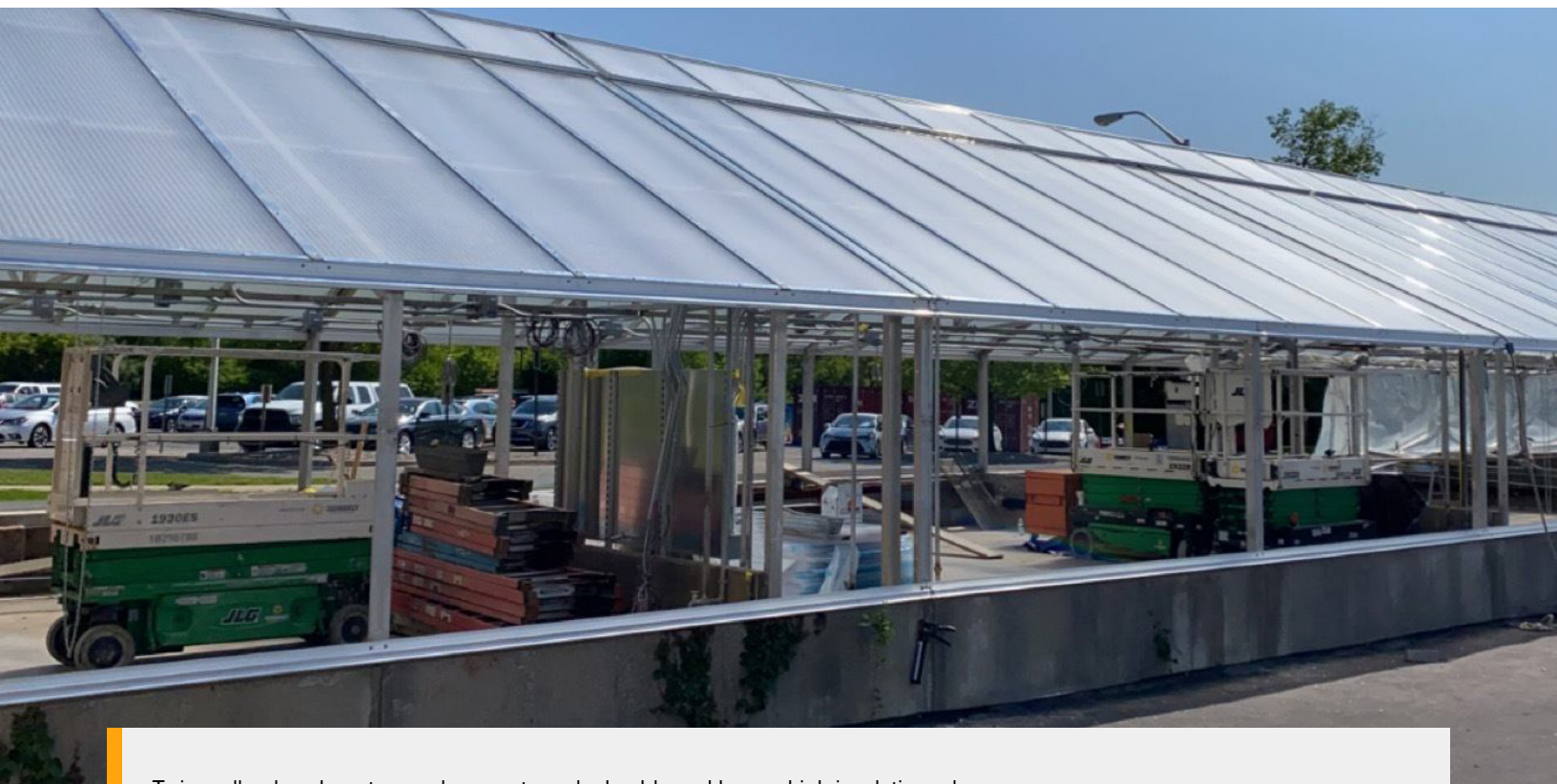
Twin-wall polycarbonate panels are extremely durable and have a high insulative value.
